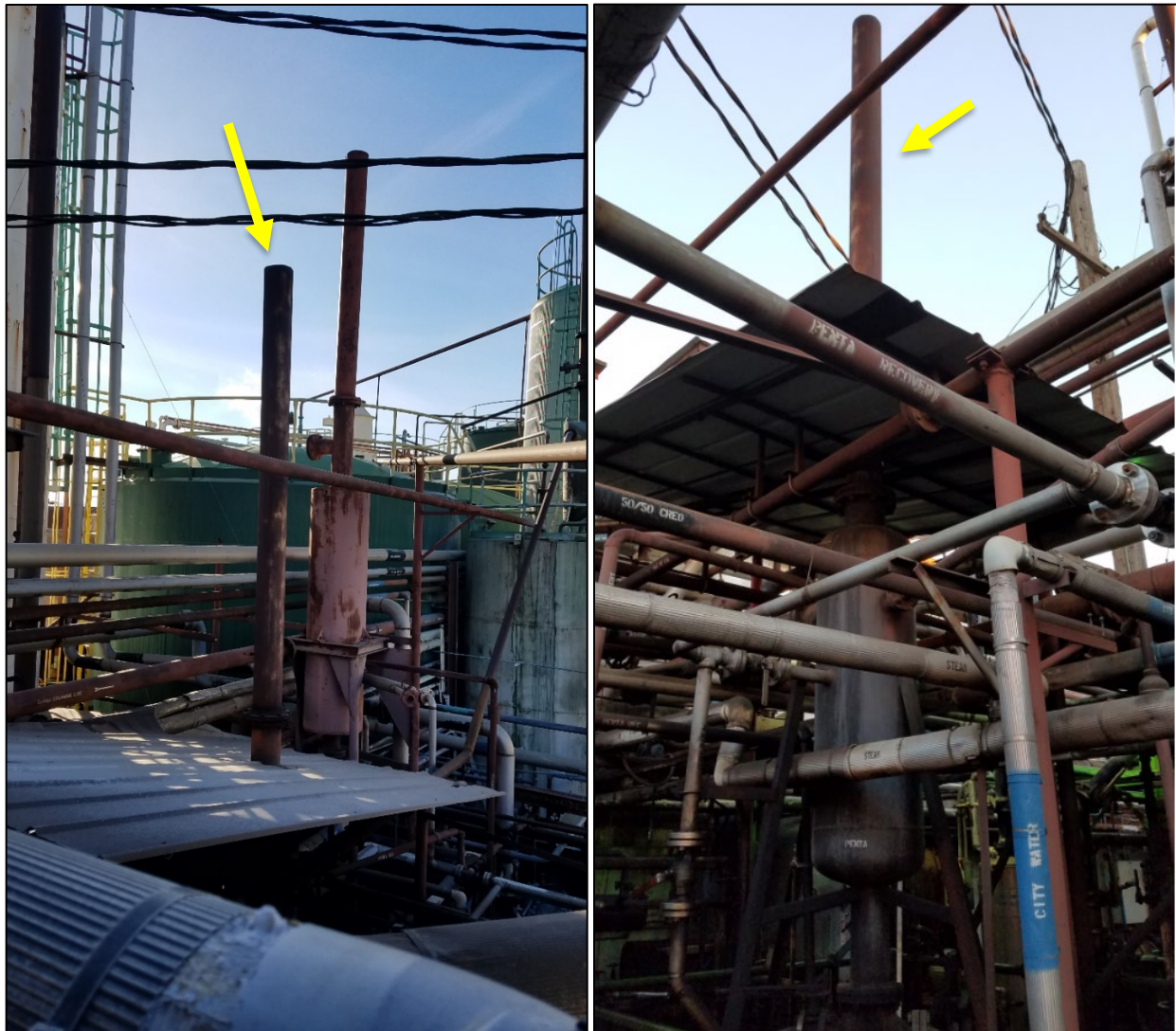
Figure 3: PCP Outlet and Sampling Location
