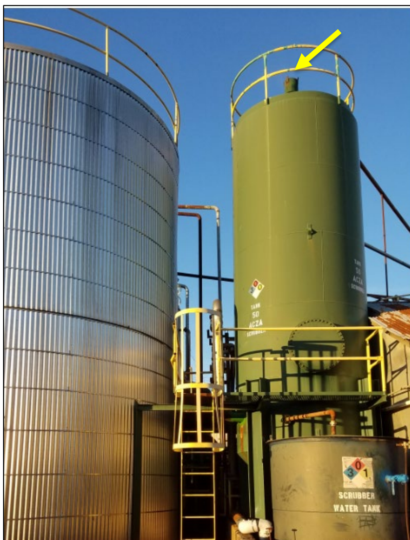
Figure 1: ACZA Scrubber Stack and Sampling Location
