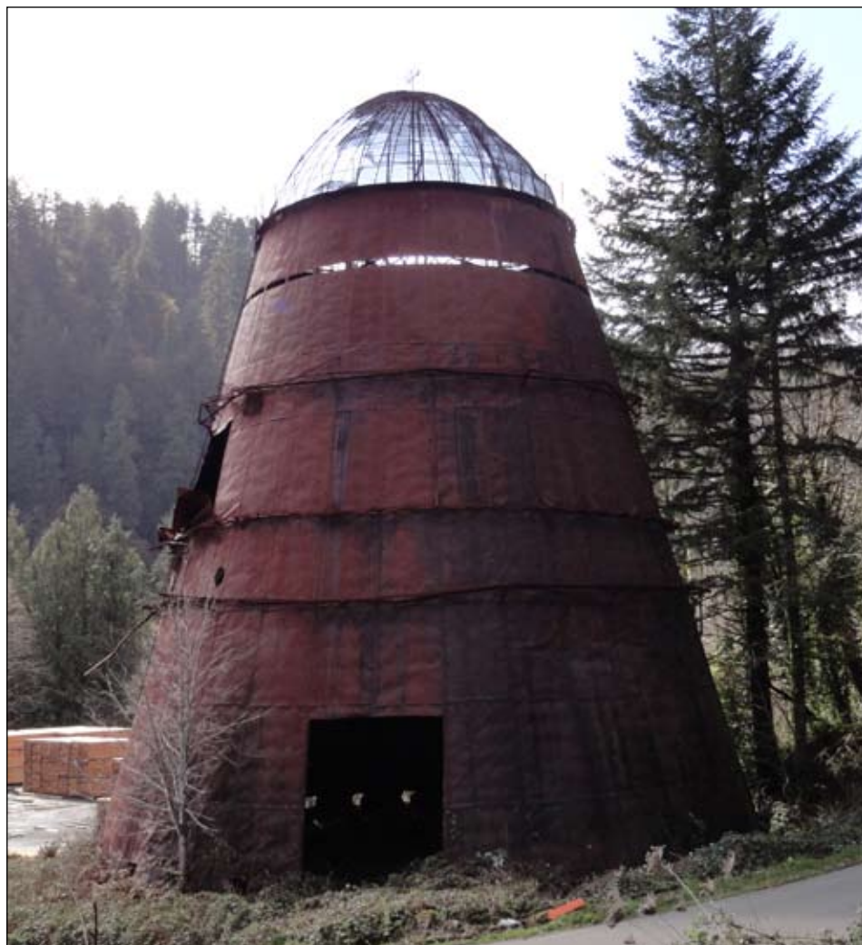
A relic from the past: Wigwam burners disappeared from the landscape as wood waste became a marketable material that could be used to make particle board, charcoal briquettes, and used as raw material for pulp and paper production. The last of the wigwam burners ended operation in the 1980's.
